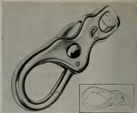
New self-locking device for hooks designed by W. H. Foster of Los Angeles.
